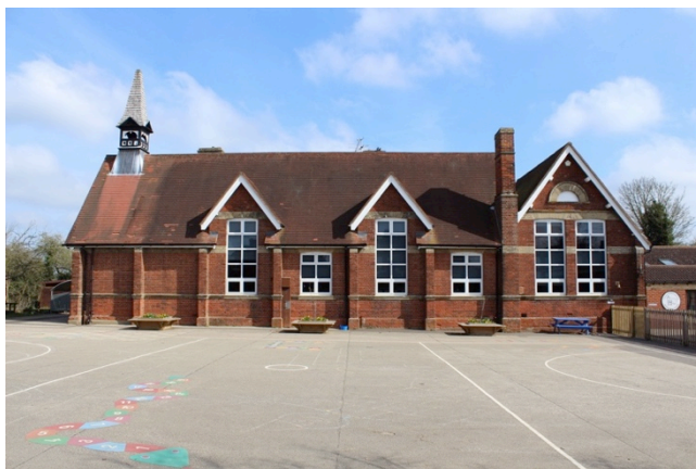
Woolpit Primary School (bell tower)
