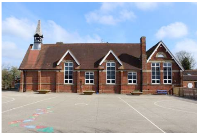
Woolpit Primary School (bell tower)
